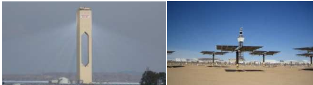
Figura 6: Central comercial “PS10” (11 MW) y central experimental “Solar Two” (10 MW)
